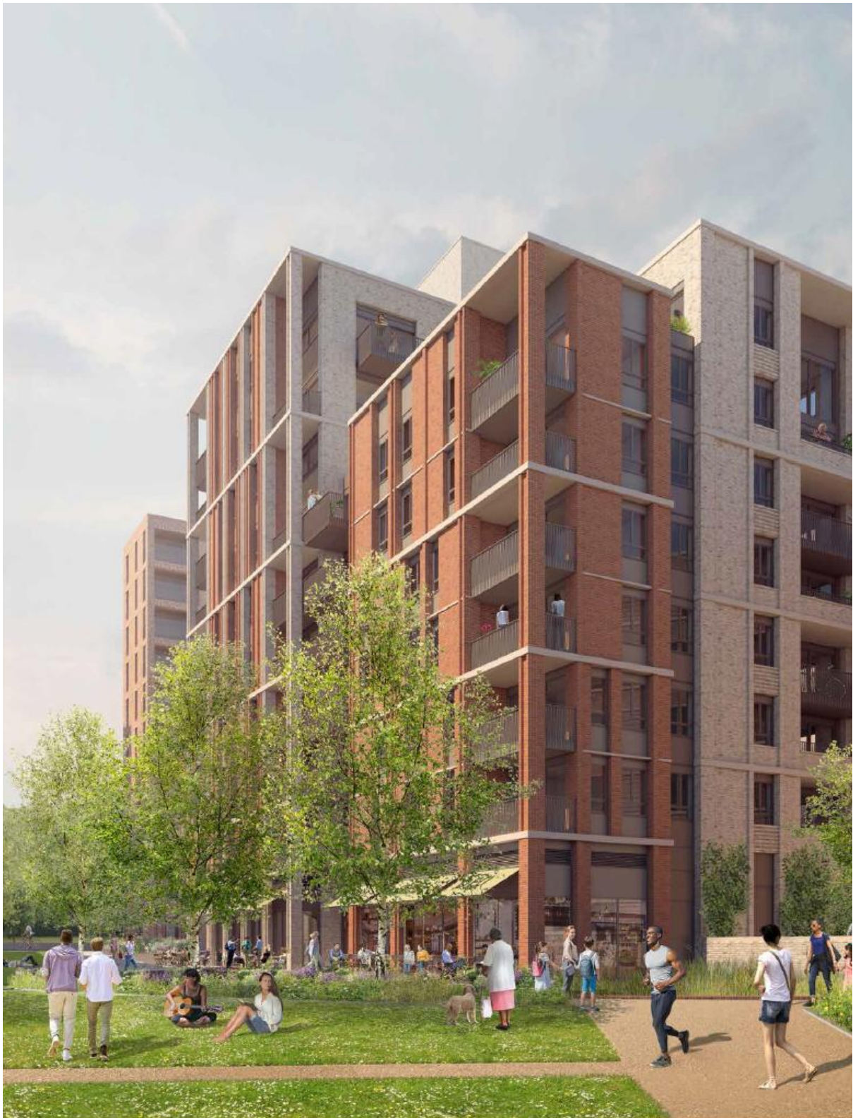
View from new Community Park looking across towards ground floor café.
